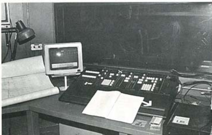
The Strand Gemini in the control room of the Rhoda McGaw Theatre.
